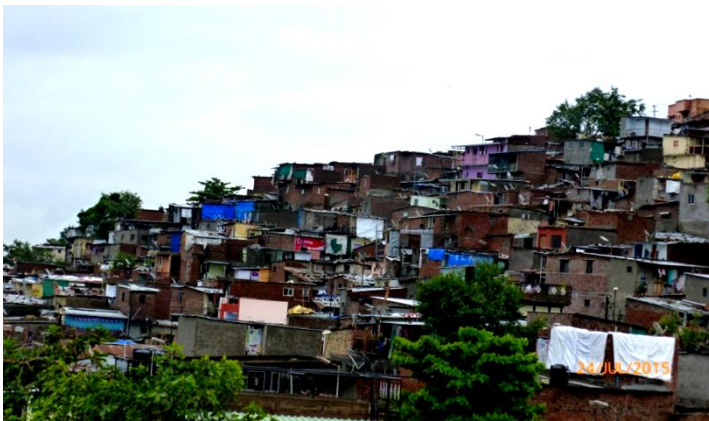
Endangering Lives - Slums Structures at Janata Vasahat Slum on Parvati Hill Slopes
